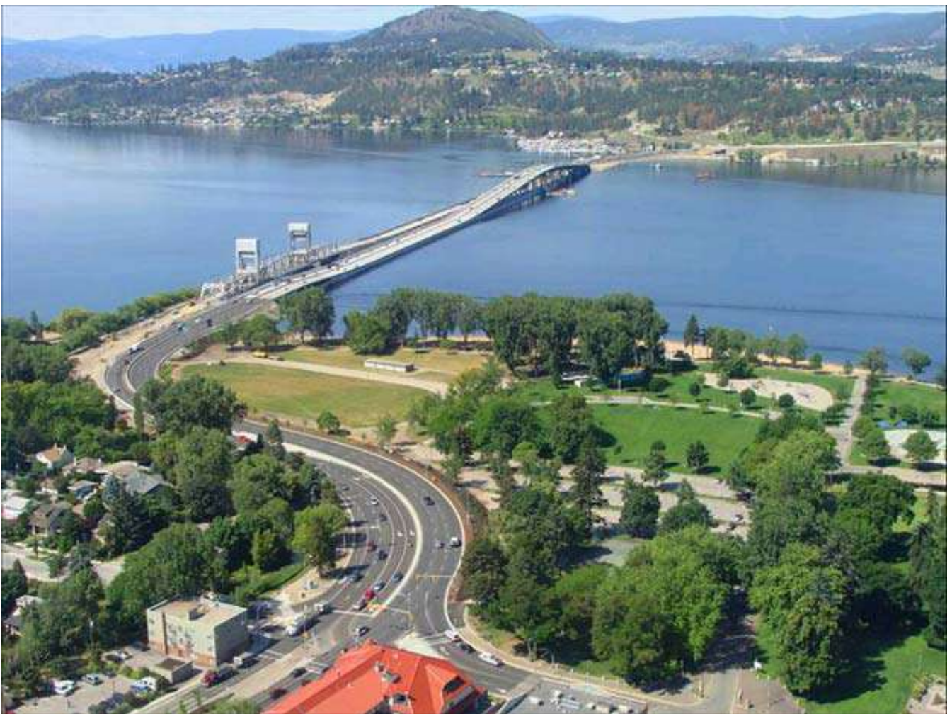
Figur 2.3: William R. Bennett Bridge, Canada
